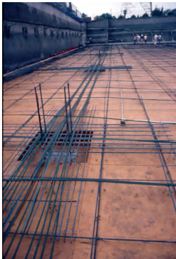
Typical Banded Tendon Layout
